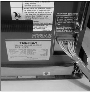
Fig. 21 Control Circuit Plug Connected to Breaker
